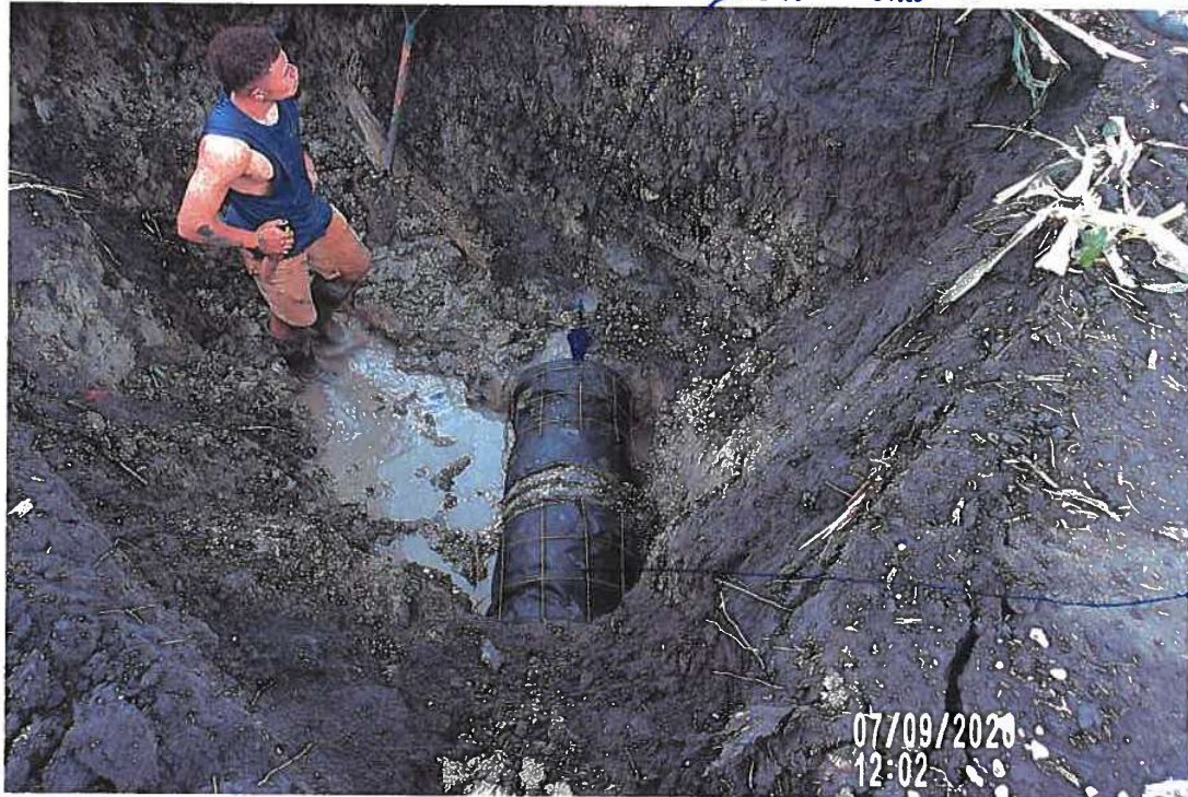
PICTURE# 4096 IS LOOKING NW SHOWING FABRIC & MESH OVER NORTH & SOUTH TIE IN JOINTS FOR 14" CLAY TILE REPAIR NORTH OF COMWAY D41
