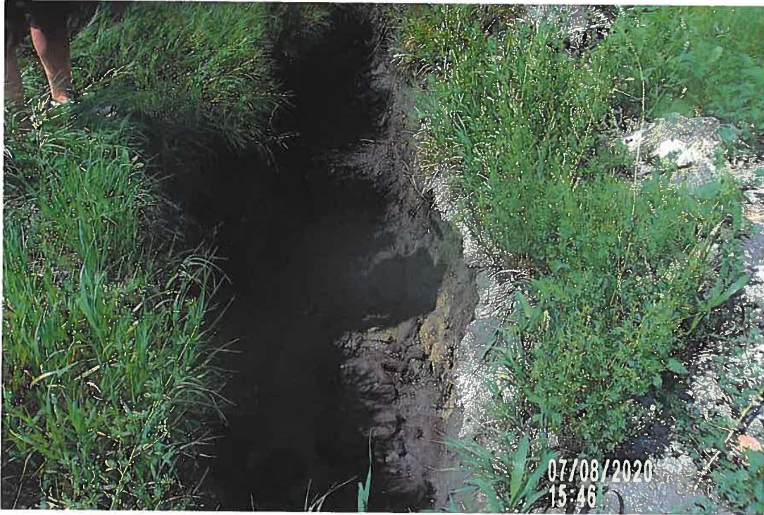
PICTURE#4067 IS LOOKING NORTH SHOWING PREVIOUSLY EXCAVATED HOLE EAST OF EAST ROW FENCE FOR CO. HWY 527 & SOUTH OF CO HWY D41
