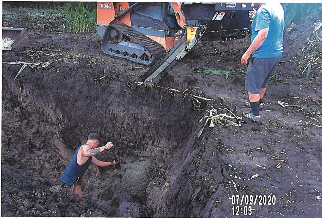
PICTURE# 4097 IS LOOK NW SHOWING CREW POURING 3/4 CONCRETE COLLARS FOR 14" CLAY TILE REPAIR FROM QUIKRETE BAGS MIXED IN A CONCRETE MIXER THAT ATTACHES TO A SKIDLOADER.
