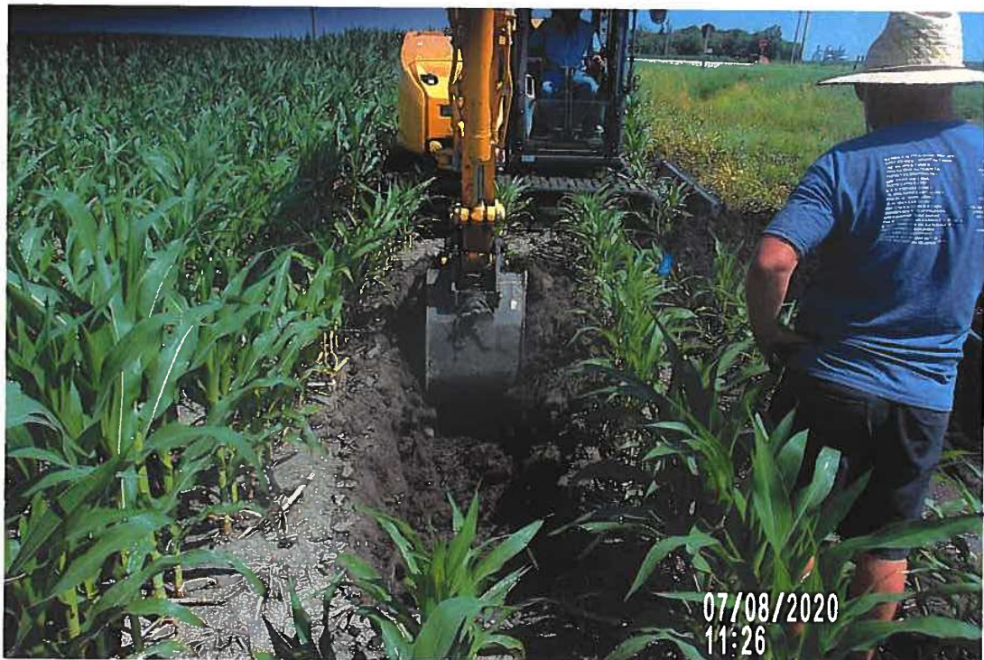
PICTURE # 4059 IS LOOKING NORTH SHOWING CREW NOW EXCAVATING ON WEST SIDE OF WATER MAIN TO CHECK IF WATER MAIN IS THE CAUSE.
