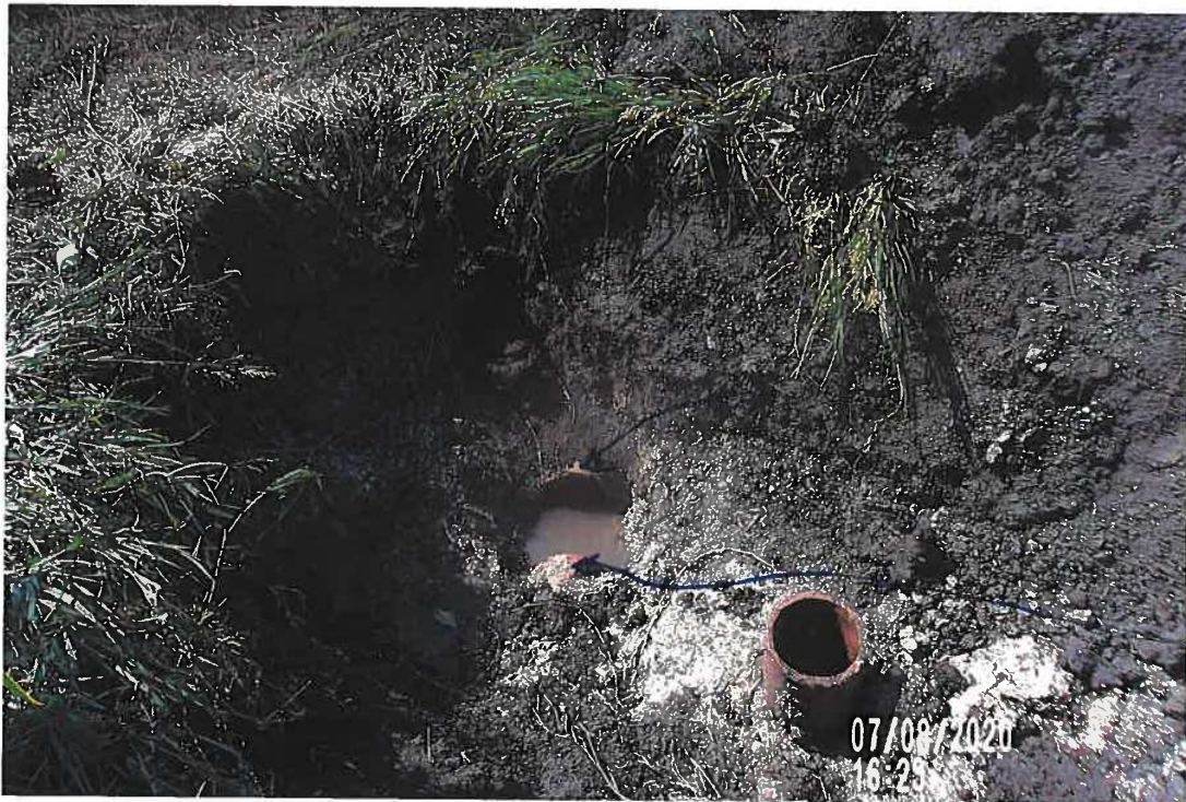
PICTURE# 4068 IS LOOKING NW SHOWING TILE FLOWING IN SOUTH DITCH OF CO HWY D41
